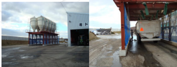
The bin approach – all concentrates in bins. Extended spouts with shade cloth on the walls. Advantage – look at all of the wasted feed (!) Disadvantage – pay more for auger delivery
