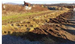
Hutches are removed
